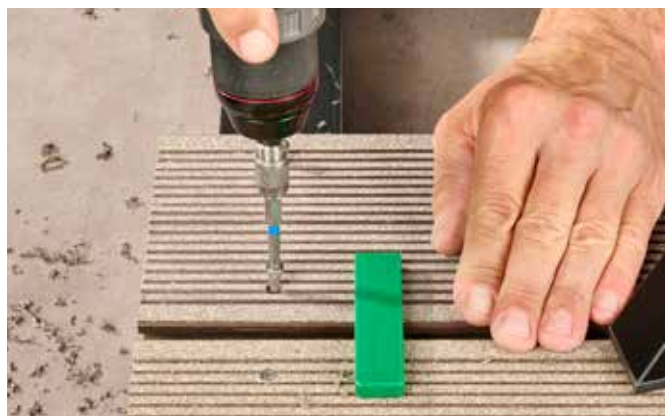
3. Screwing the decking board in place
