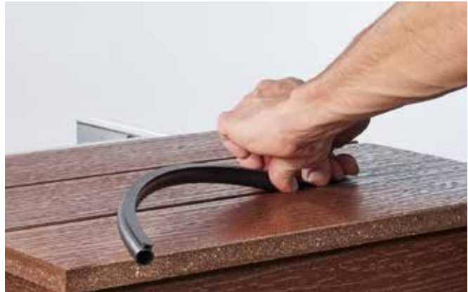
Manual installation by pushing
