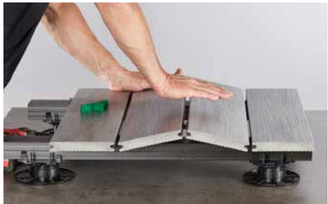
2. Inserting the boards
