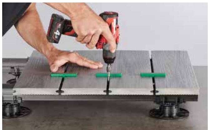
3. Screwing down the Installation Clips again
