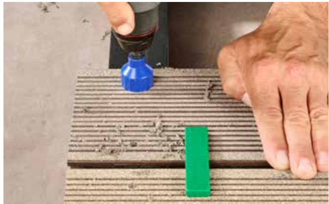
2. Drilling and countersinking
