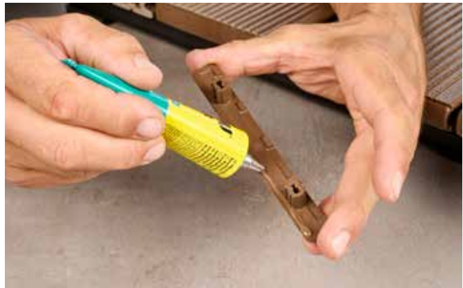
1. Applying glue to the upper edge side
